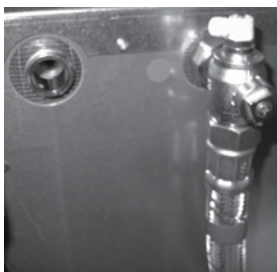
Heating circuit outlet (forward flow) connection
